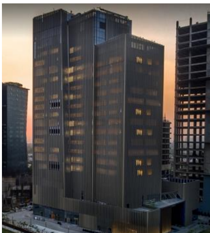
Max Towers, Noida Status - Completed
