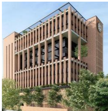
Max House Okhla Phase 1 Status – Completed
